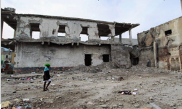
PAP school devastated by the 2010 earthquake
